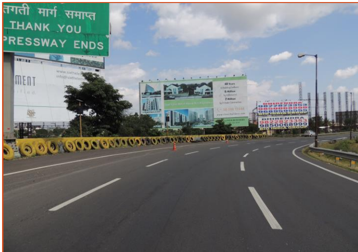
End of Expressway - Towards Pune
